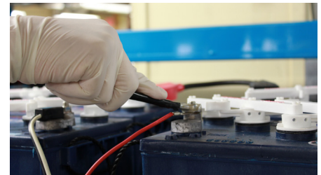
Figure 8: Reattach positive lead to the positive terminal after disconnecting AC power.
