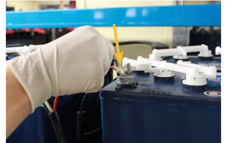
Figure 7: Touch the positive lead to the positive terminal for 3 seconds
